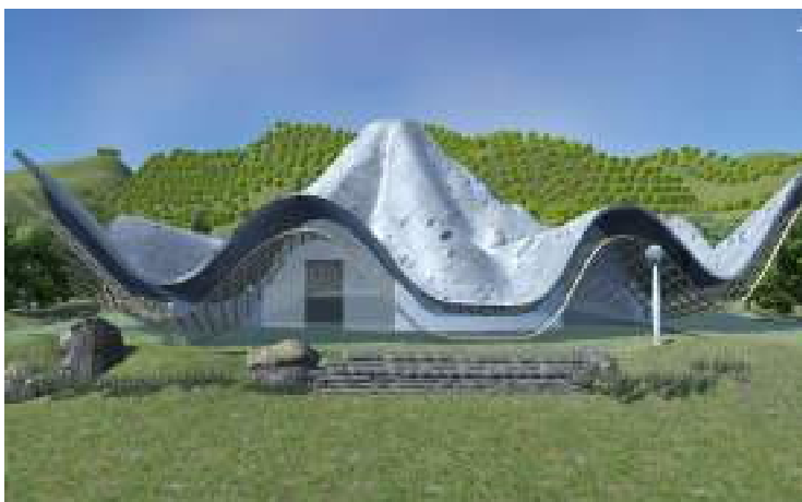
Geometry clashing after optimisation – bamboo substructure and concrete shell
